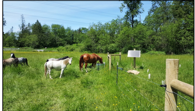
Solar Powered Pump, an example of SCD's Technical Assistance
