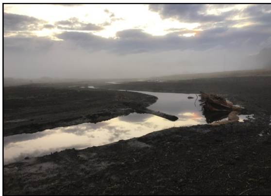
Trumpeter Creek Restoration project. Skagit County partnered with the Skagit Land Trust and Ducks Unlimited.
