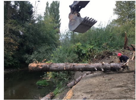
Installing Large Woody Debris for bank stabilization and fish habitat
